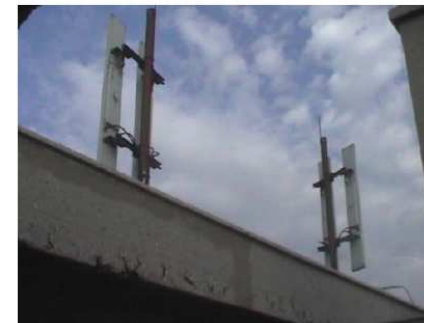
FIG: Example with roof-top antenna system in sectorial arrangement mounted at a height of 48 m above ground. A view to the 2 sector of base station antenna system. The radiated power per channel is P=955 W at 935 MHz.
